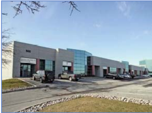
Bonhill Road Mississauga
