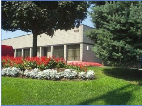
Meyerside Drive Mississauga
