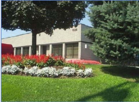
Meyerside Drive Mississauga
