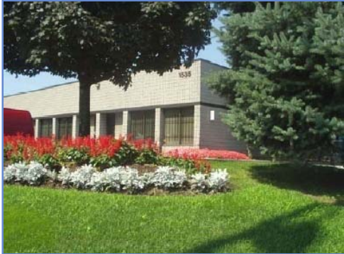
Meyerside Drive Mississauga
