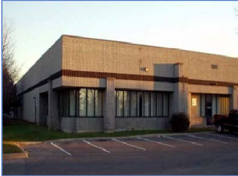
Courtneypark Drive Mississauga
