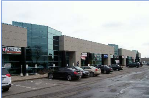
Dixie Road Mississauga
