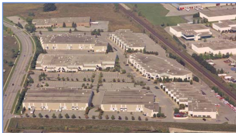
Millcreek Business Centre III
