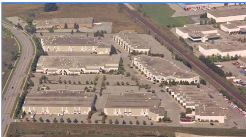
Millcreek Business Centre I
